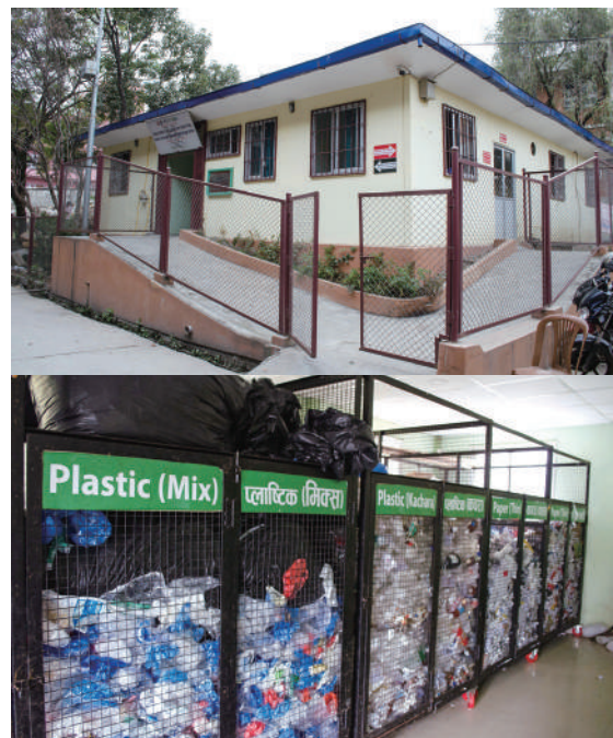
Figure 13: The waste treatment centre (top) and Storage for recyclable wastes (bottom) (Source: HECAF 360)
